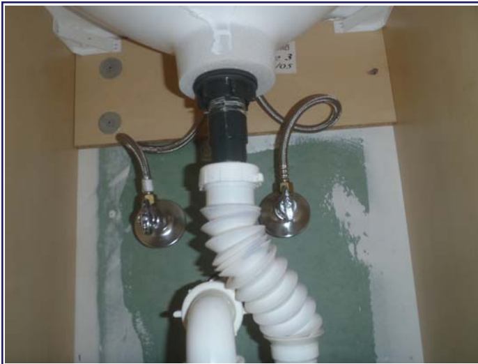
Flexible drain line installed below the bathroom sinks
